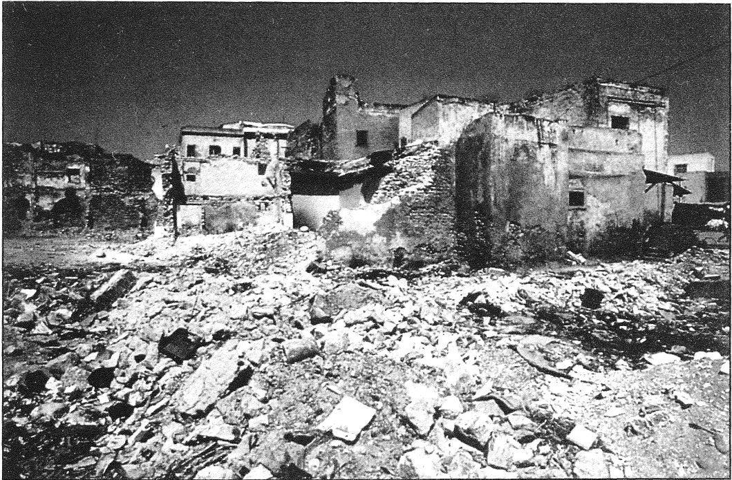
Dilapidated and demolished buildings in Hafsia, before project.
