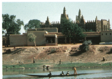
Figure 13 In this award-winning design for a health clinic in Mopti, Mali, it is clear that the new (structure in front) can be harmoniously integrated with the old (structure in back) without breaking the code.
